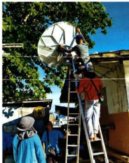
Installing an antenna to use CONNECTme NOW's satellite broadband
